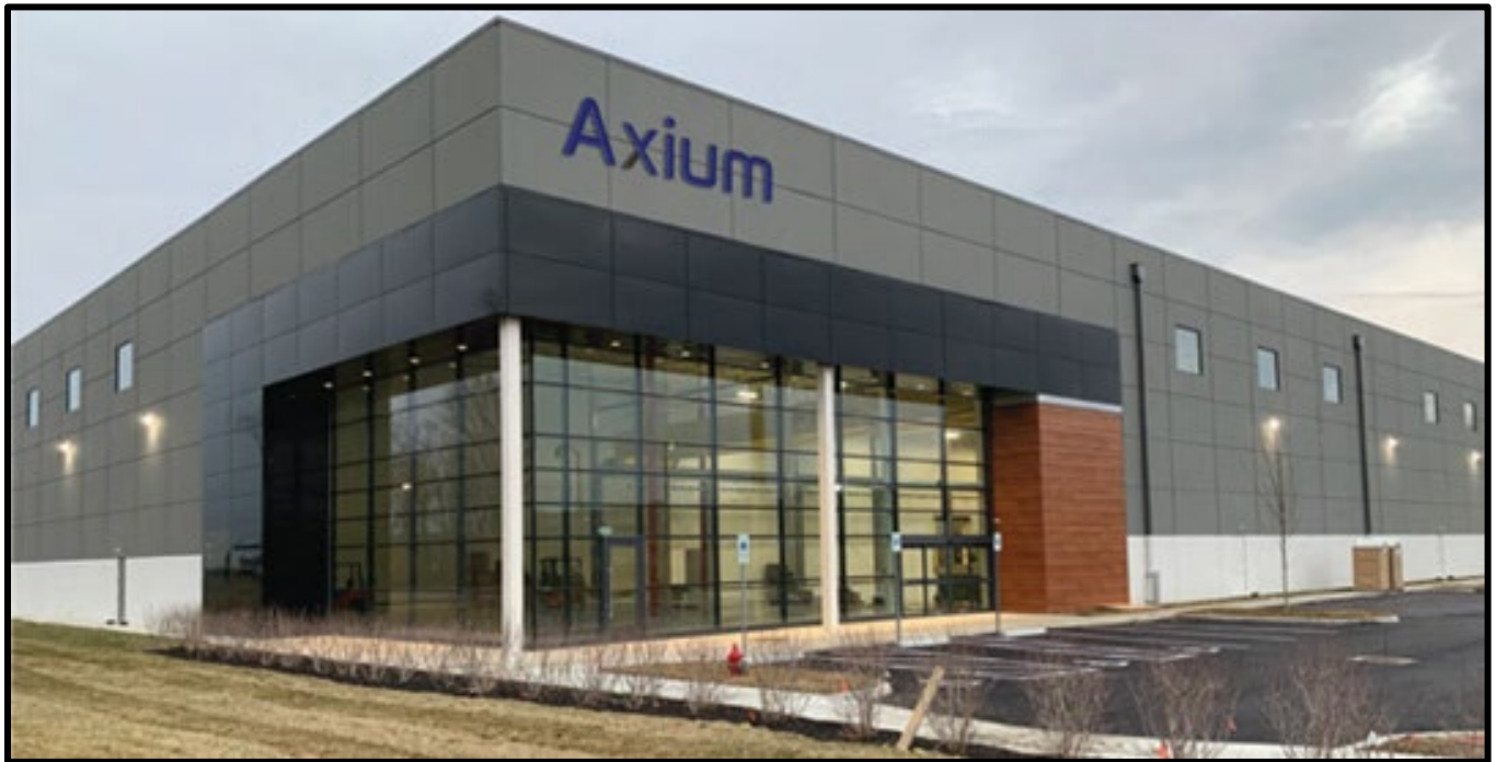
Axium's Bartlett, Illinois Plant
